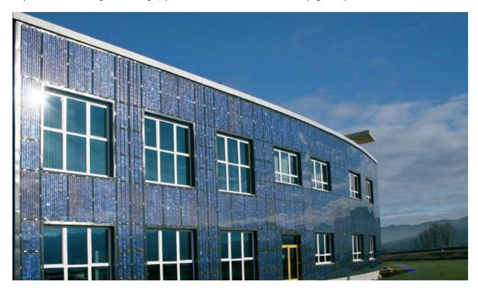
Solar Innova modules integrated photovoltaic technology used in the BIPV installations are multifunctional. That is, in addition to generating electricity, also meet all the requirements demanded by conventional facades weather protection and acoustic agents, heat insulation. On the other hand, represent an innovation aesthetic character regarding conventional facades.
