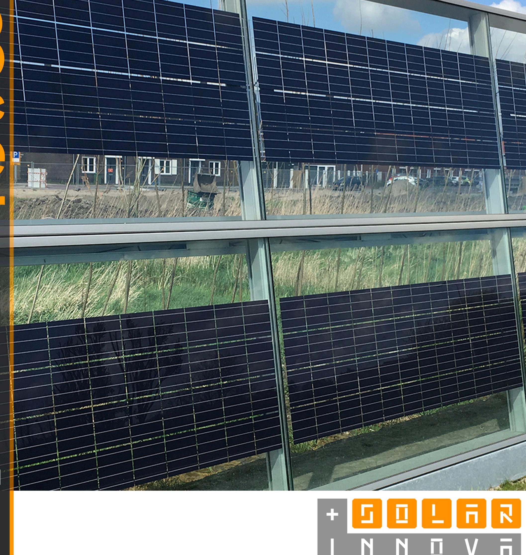
hotovoltaic noise barriers are physical obstructions with BIPV panels designed to produce renewable energy and also reduce the noise level between noise sources and places like hospitals, schools and residential areas ...
