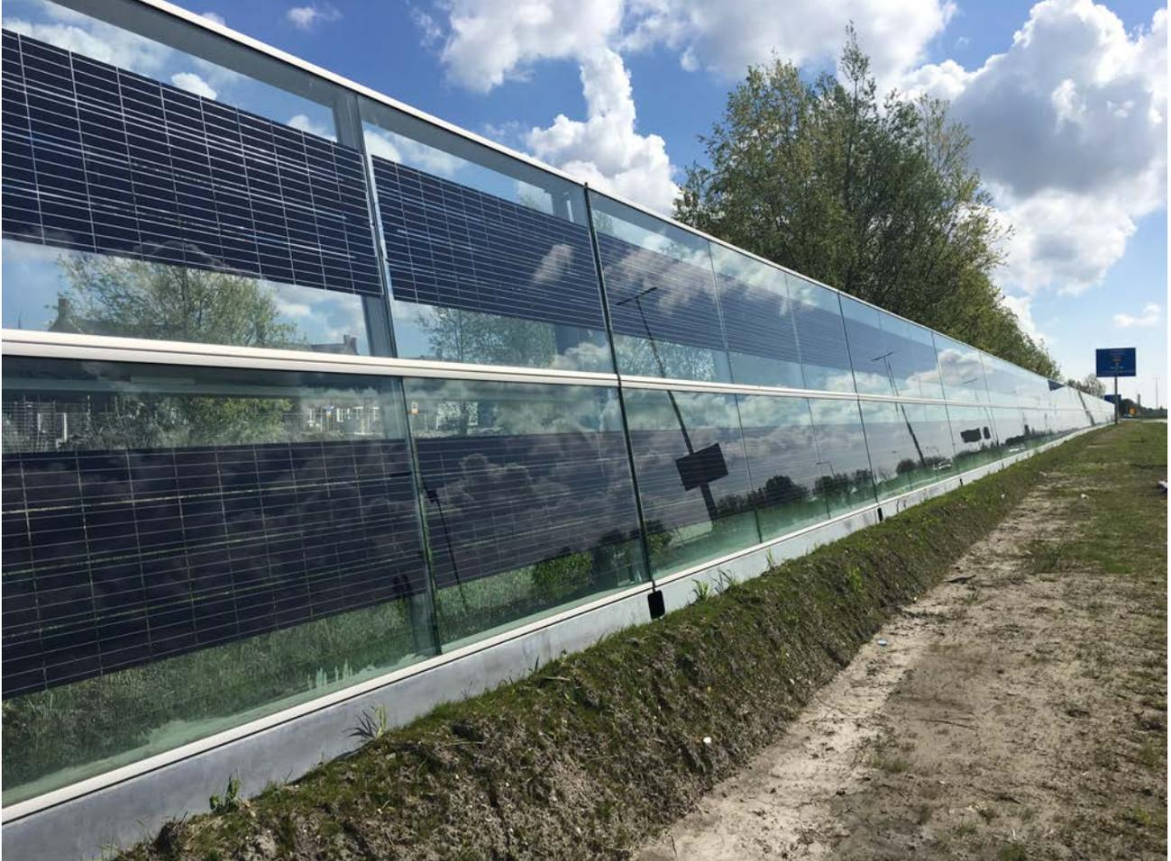
PhotoVoltaic Noise Barriers are physical obstructions with photovoltaic panels designed to produce renewable energy and also to lower noise levels between noise sources and sensitive receptors, such as hospitals, schools and residential areas.
