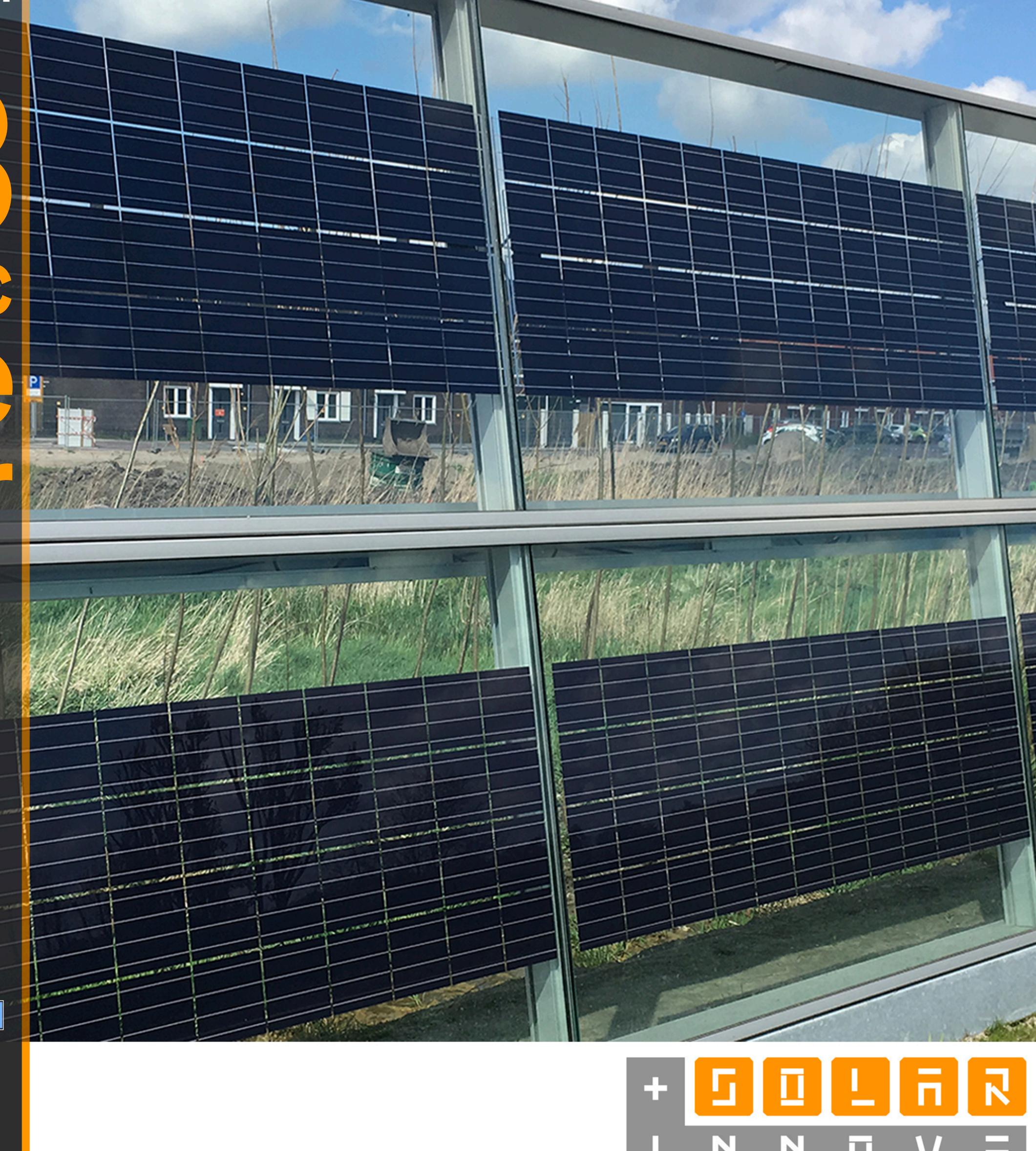
Photovoltaic noise barriers are physical obstructions with BIPV panels designed to produce renewable energy and also
