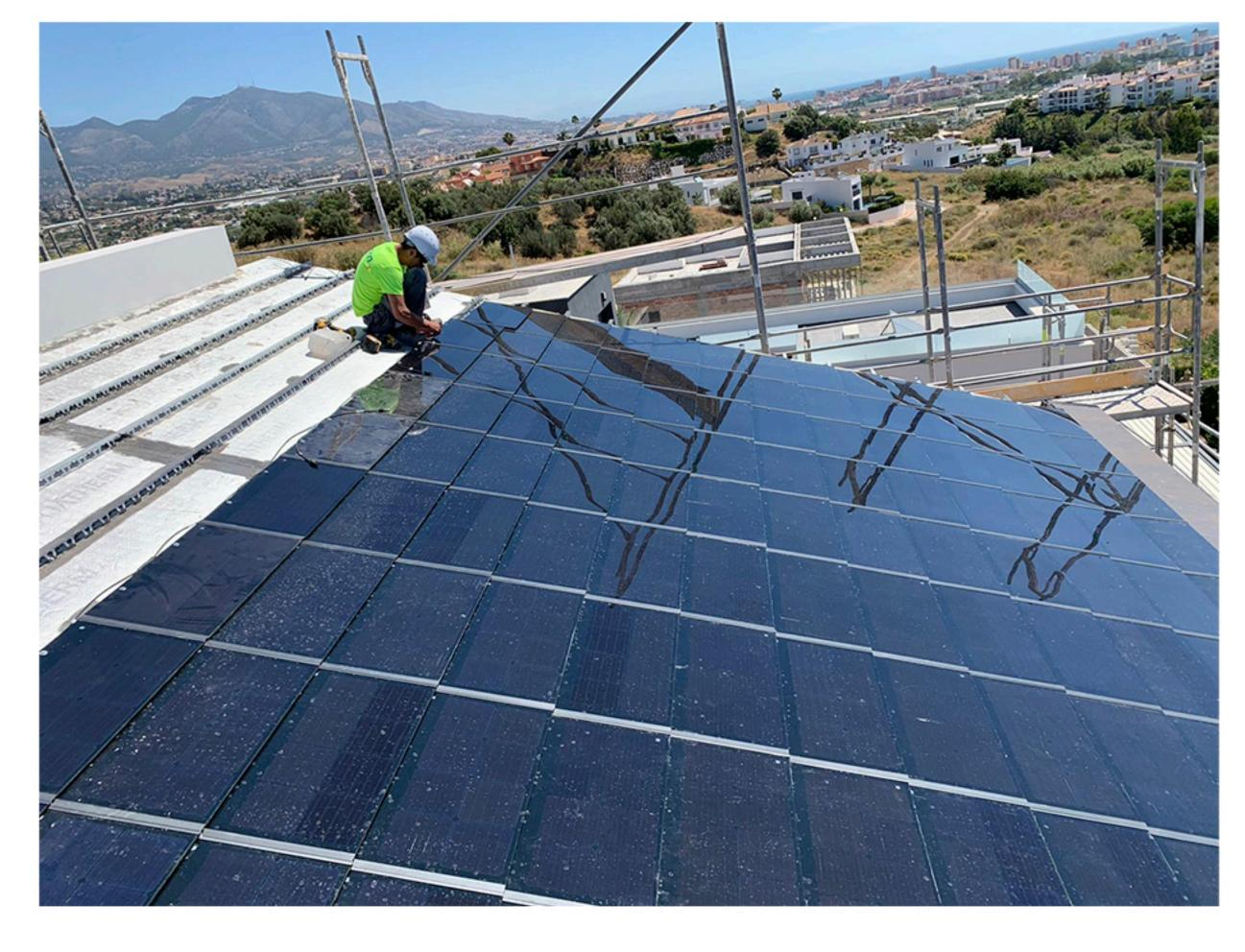
Solar roof tiles are a perfect solution by constituting an active technological glass range being able to produce electrical energy, used on new bulidings and refurbishment.
