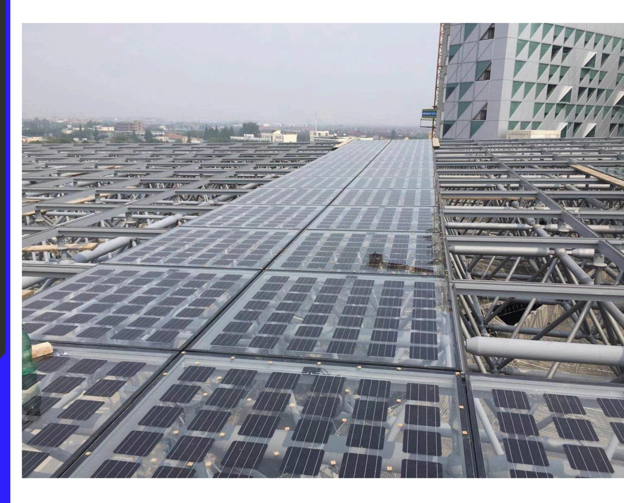
ne of the great advantages of Solar Innova's architectural integration photovoltaic glasses is that they act as a filter for ultraviolet and infrared radiation, both harmful to health, in addition to generating clean and free energy thanks to the sun.
