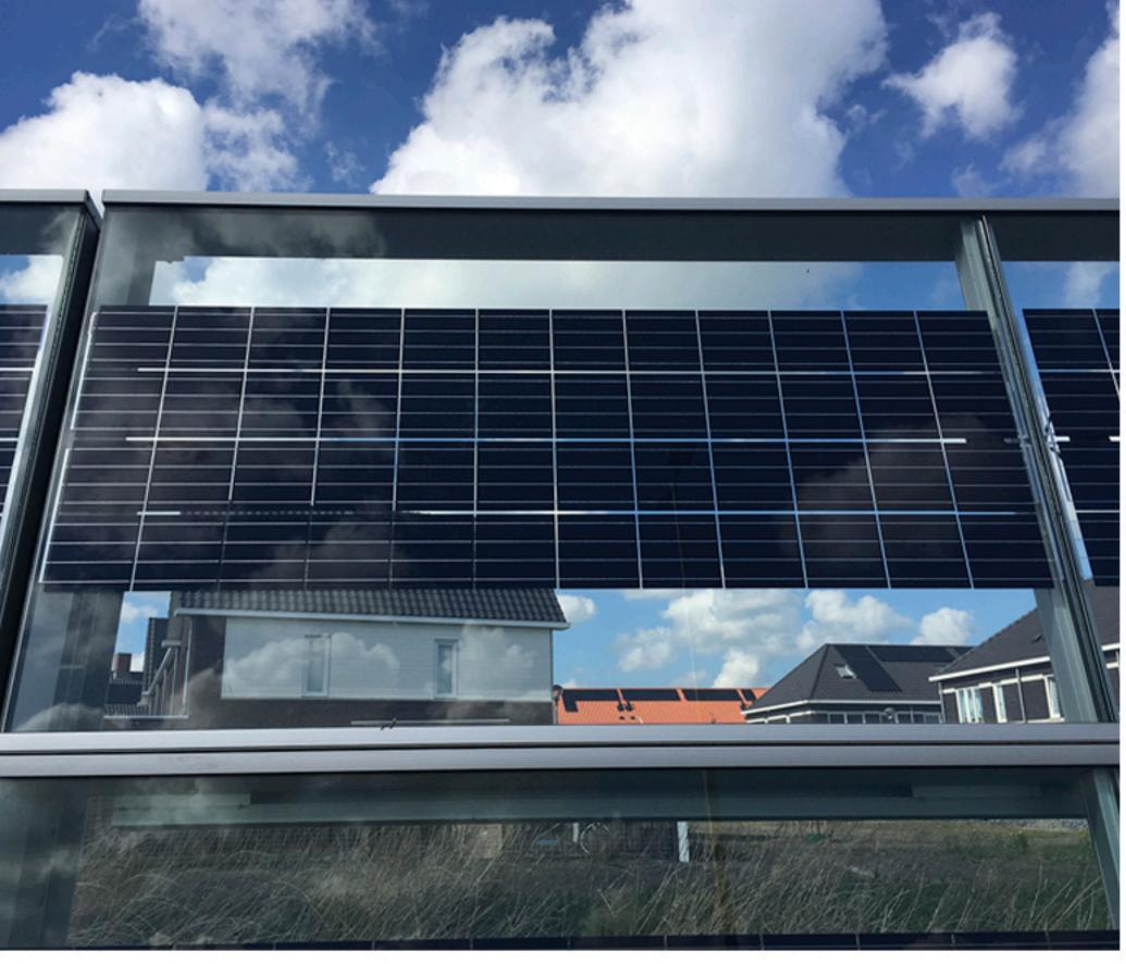
hotovoltaic noise barriers are physical obstructions with BIPV panels designed to produce renewable energy and also reduce the noise level between noise sources and places like hospitals, schools and residential areas ...
