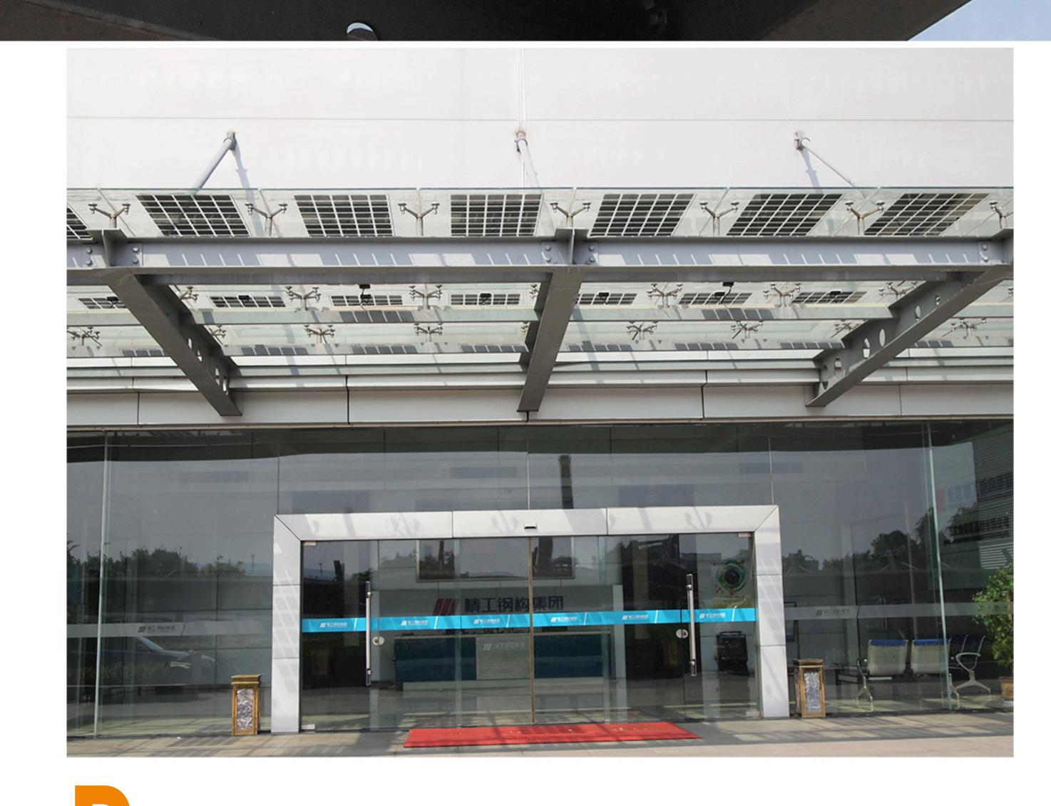
hotovoltaic facades are an alternative way to transform materials that are normally used in construction to generate shades.
